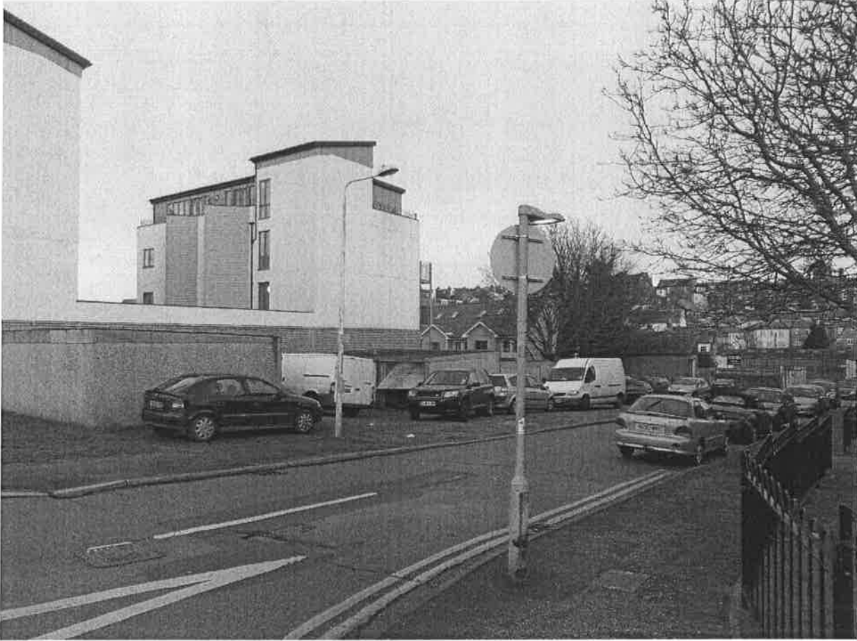
F/TH/14/0092 – Garages Adj. Pikes Lane, Sussex Street, Ramsgate
